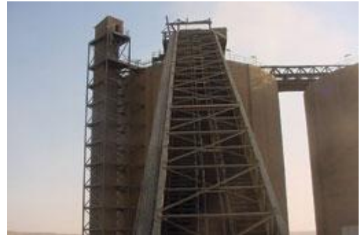
General View of Elevator Lifting Clinker Into Silos
