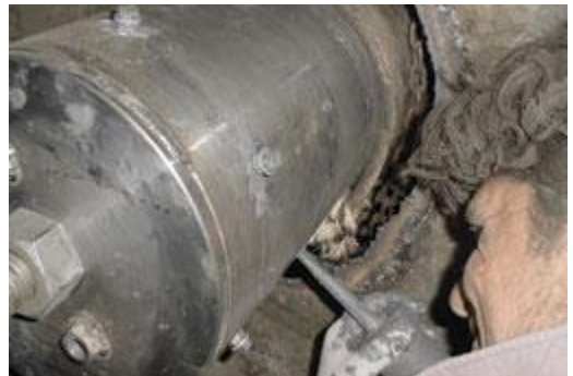
Former in place with injecting of the Belzona® 1311 (Ceramic R-Metal)
