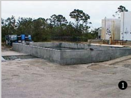
General view of the containment area.
