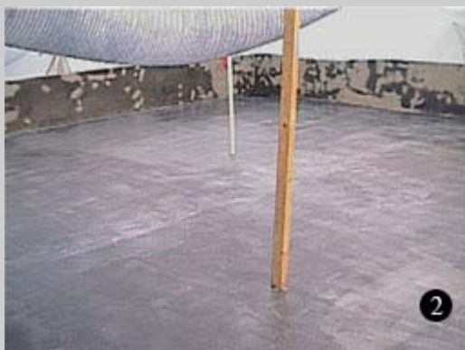
Belzona® 4911 and Belzona® 4141 applied.
