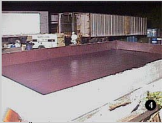
Belzona® 4311 applied over night, completing the application process.
