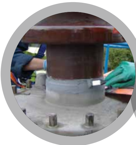
Joint Sealing
